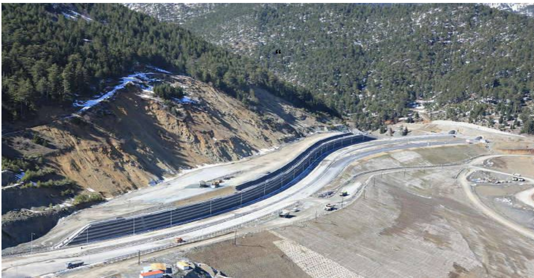
“Big Cut stabilization” in Egnatia Odos motorway - During Construction
