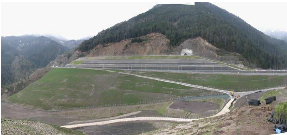
“Big Cut stabilization” in Egnatia Odos motorway - During Operation
