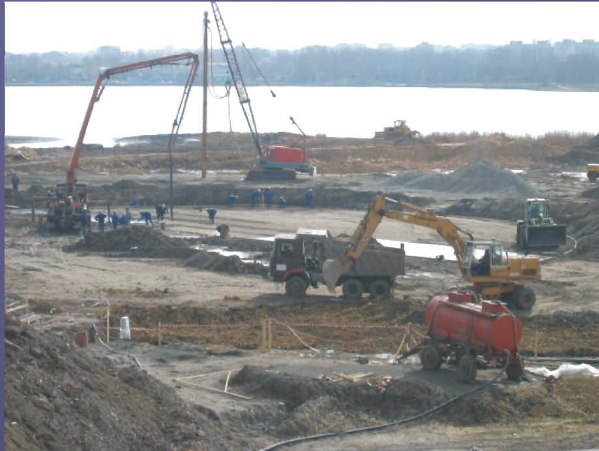
Constanta Sewerage and Wastewater Treatment - Ground improvement
