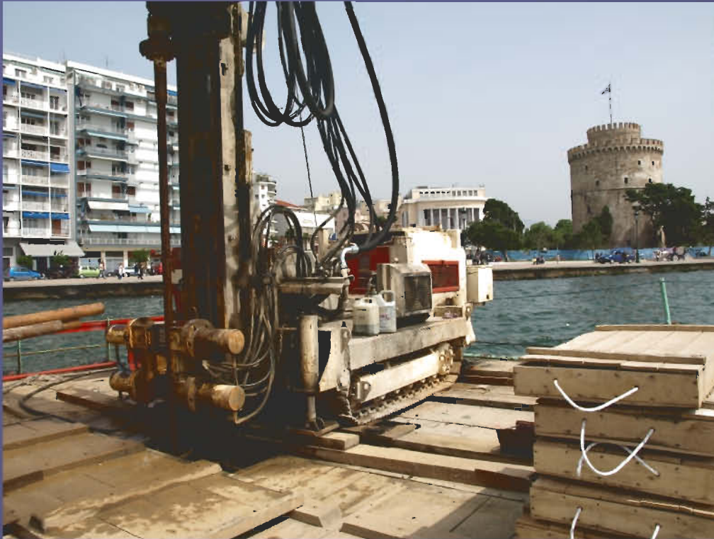
Offshore geotechnical investigations
