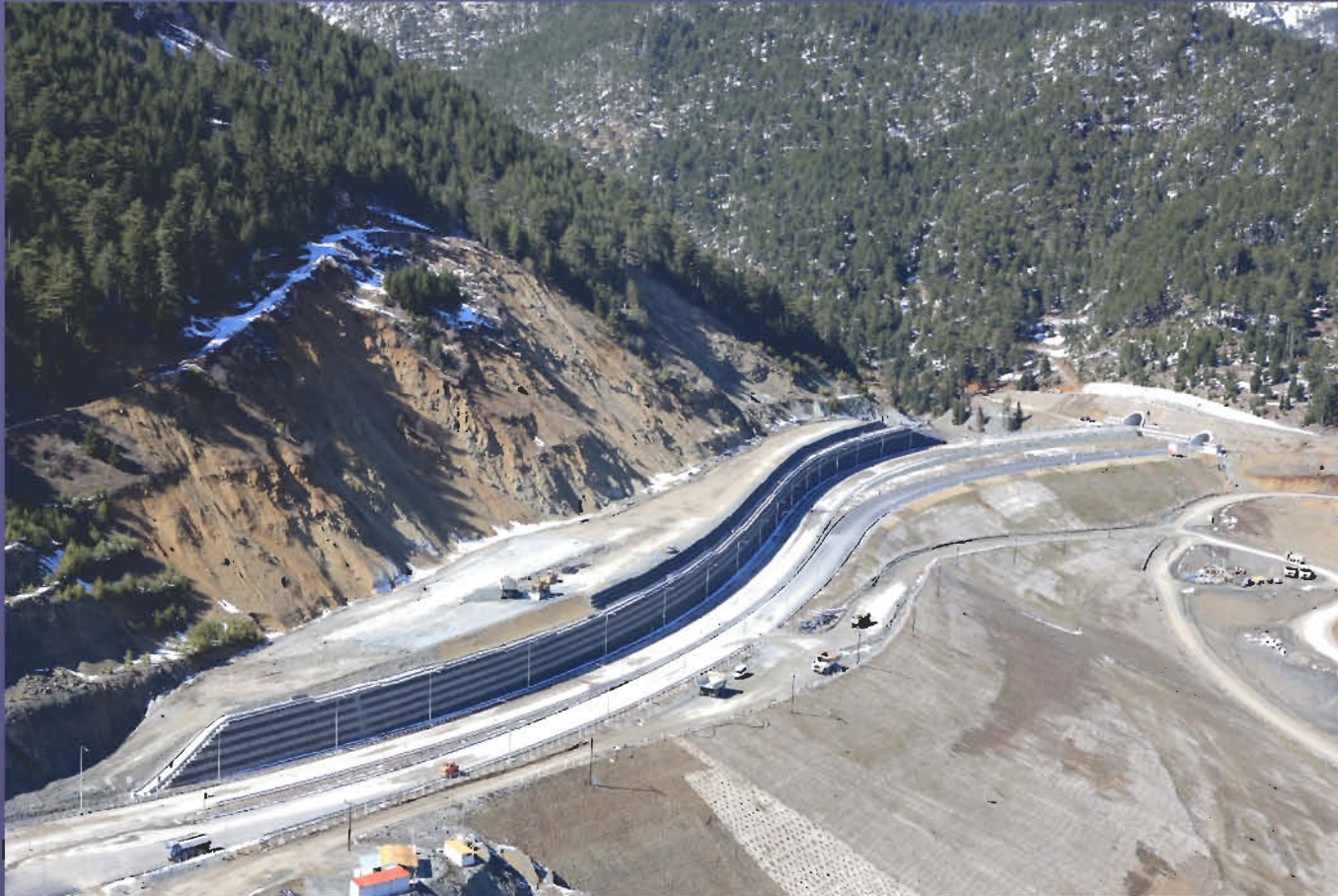
Metsovo - Landslide stabilization
