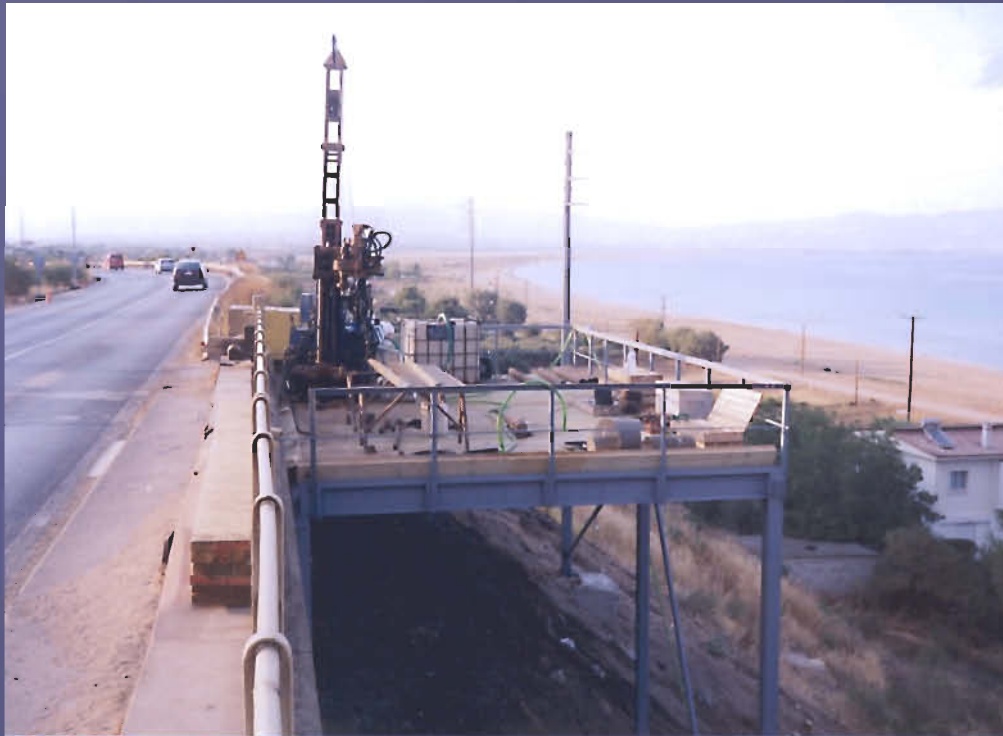
On shore geotechnical investigations
