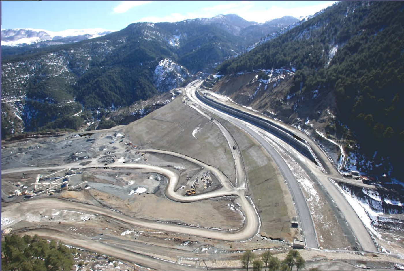
Metsovo - Landslide stabilization
