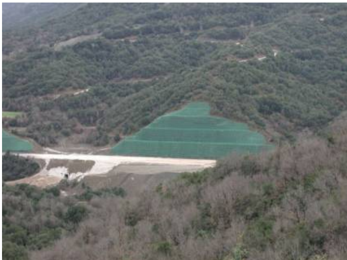
Reinforced cuts - soil nailing
