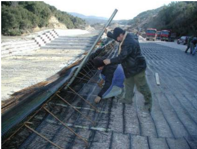
Reinforced cuts - soil nailing
