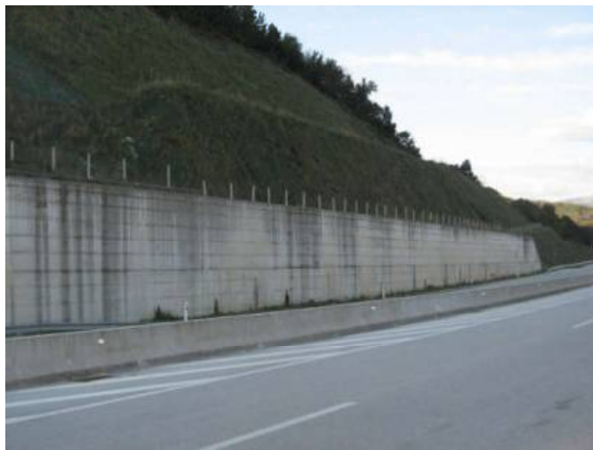
Agia Anastasia Reinforced Cuts (anchored walls and soil nailing)
